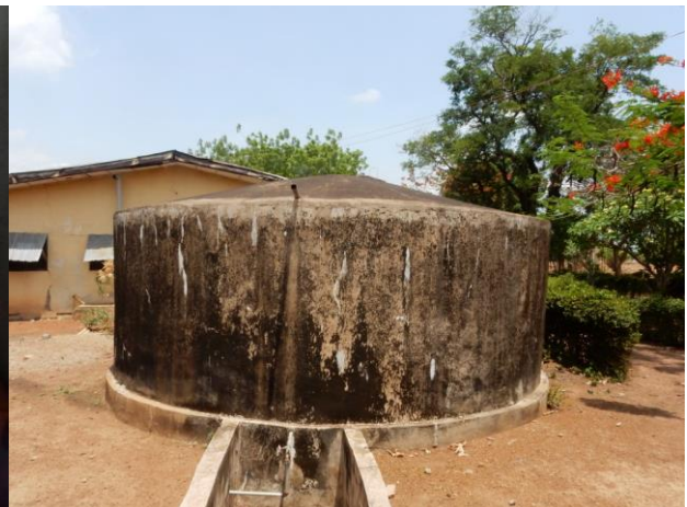
Broken water reservoir
