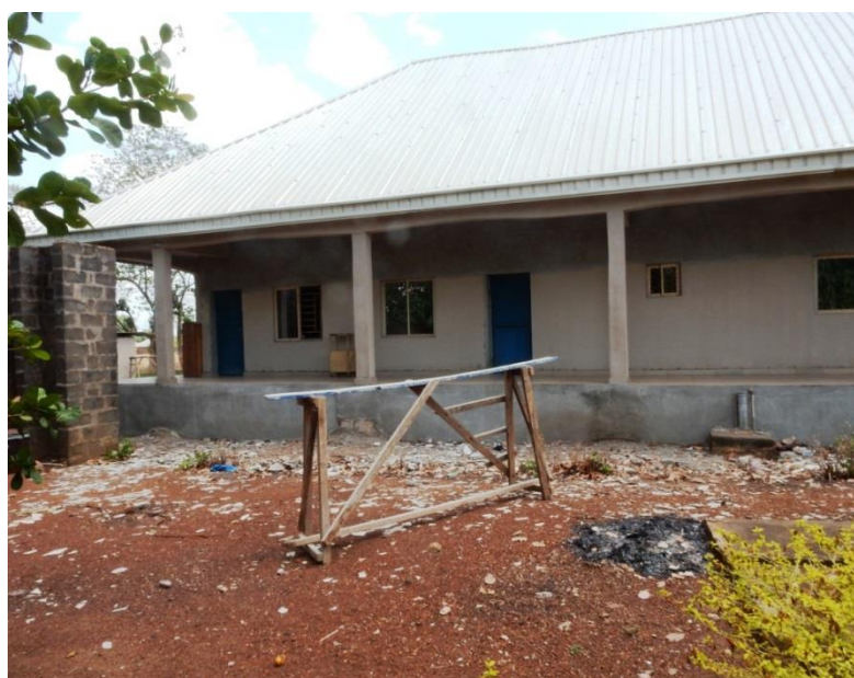
Renovation still in progress
